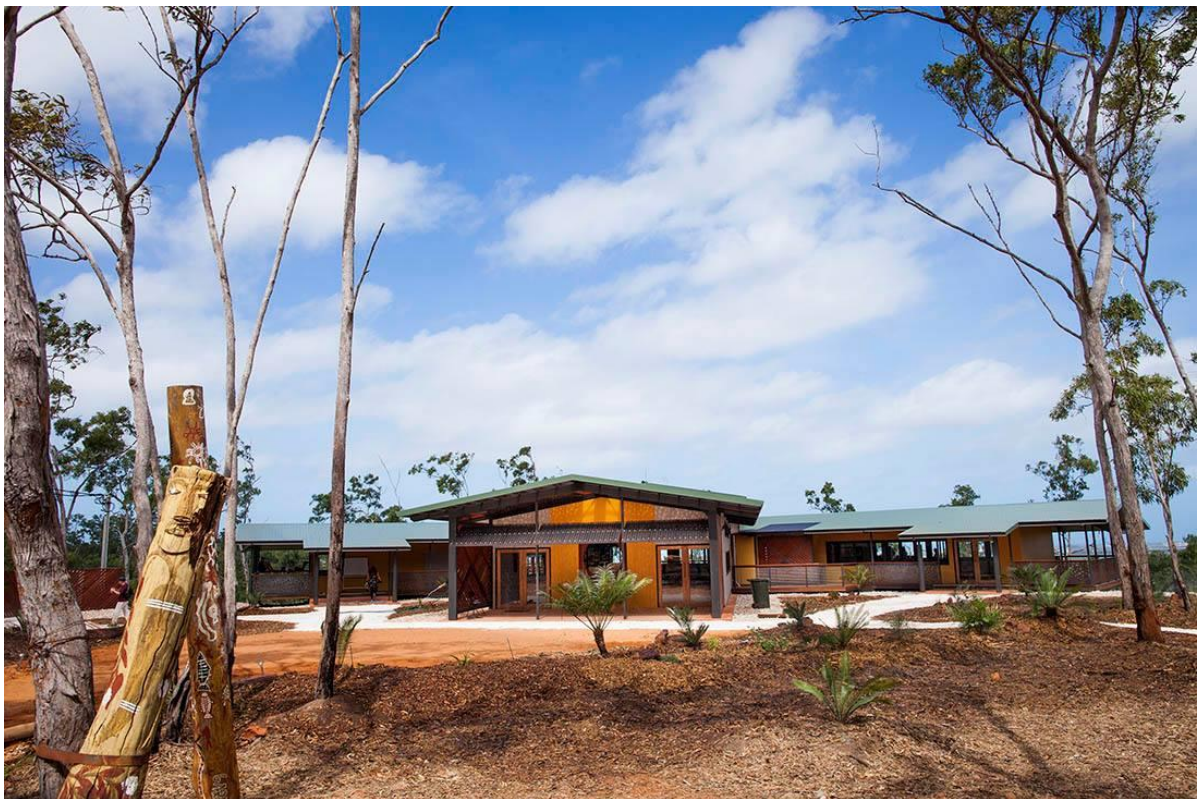
Figure 3: Frontage of the Garma Cultural Knowledge Centre showing the shank and arms of the anchor (Image: Peter Eve 2014).
