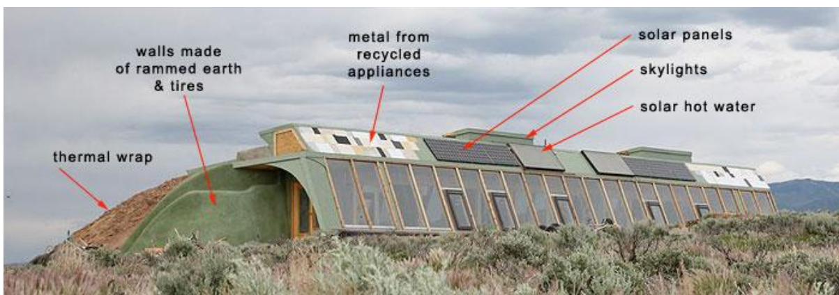
Figure 2.1 - Global Model Earthship in Taos, New Mexico, USA (Earthship Biitecture, 2012a)
