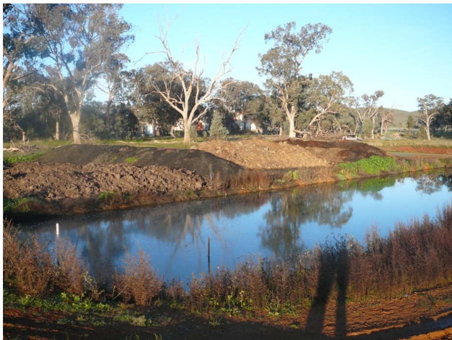
Figure 12. The settling pond for waste water treatment and marc heaps at Whitebox Winery
