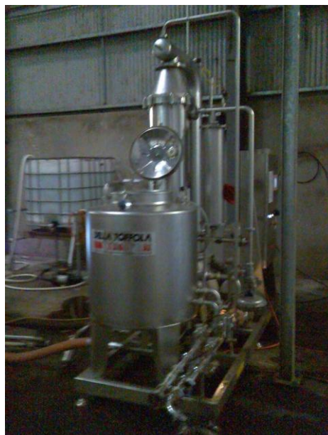
Figure 6. Cross-flow filter at Whitebox Winery
