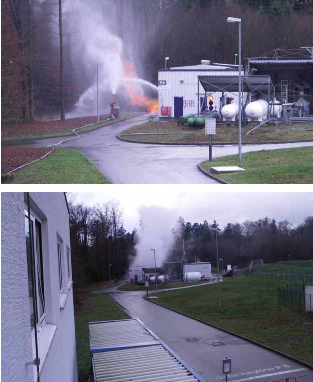
Figure 5.3: Photographs of the test cell during a BKH test run, taken from the D68 control building.
