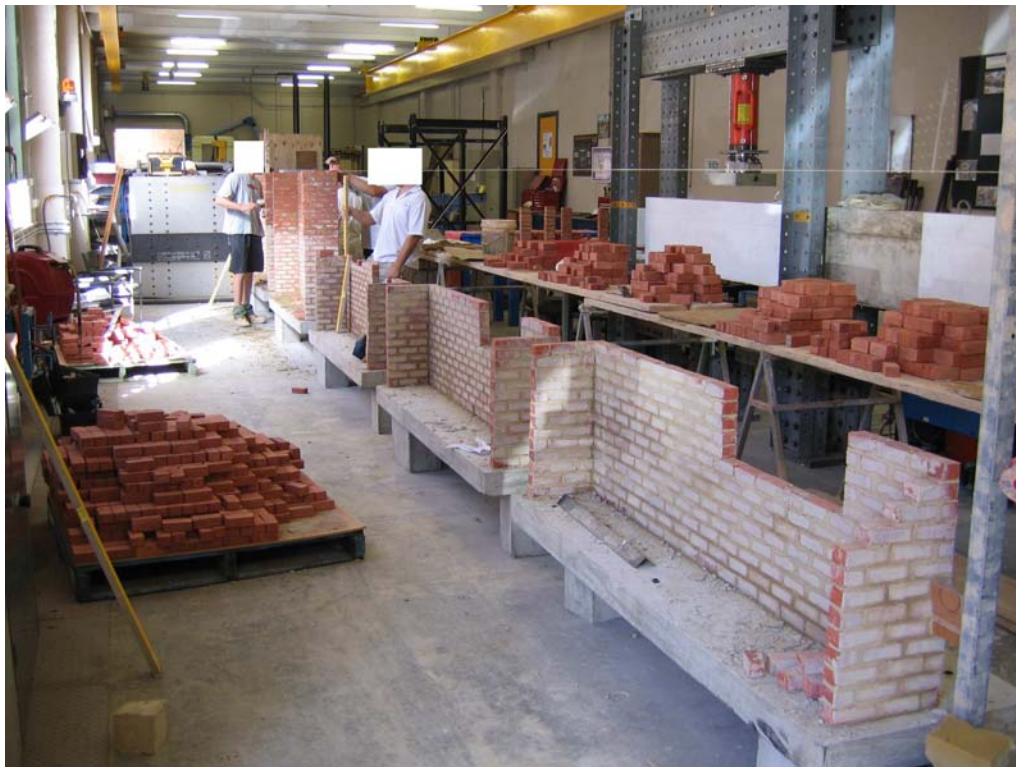
Figure 3.1: The test walls during construction.
