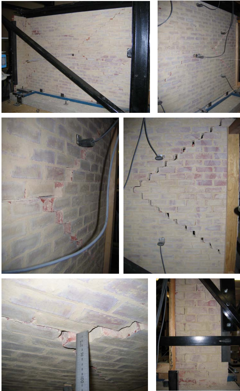
Figure 3.23: Wall D1 at the conclusion of testing.
