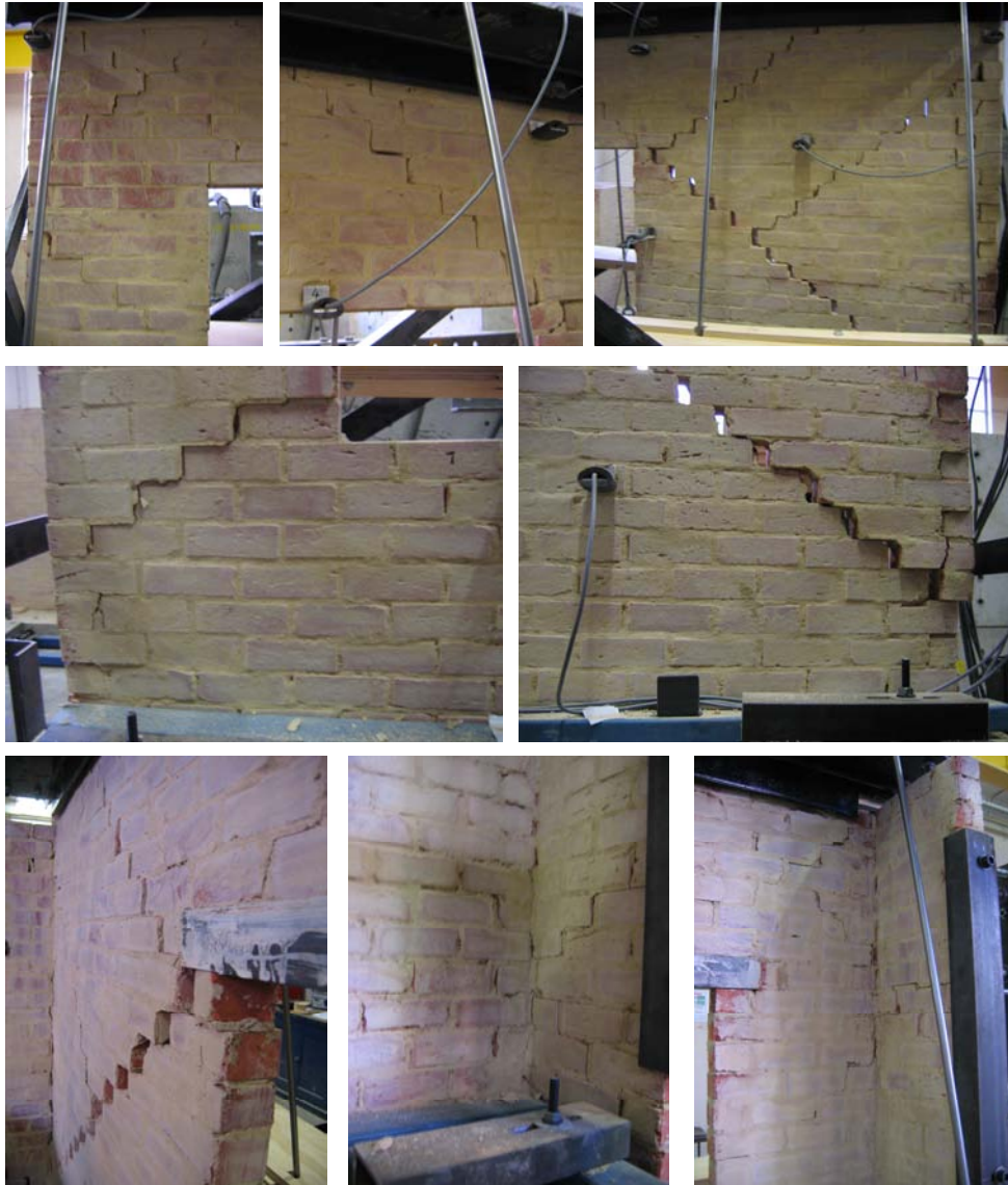
Figure 3.25: Wall D3 at the conclusion of testing.
