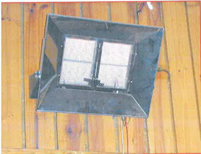
Wall mounted unflued gas heater
