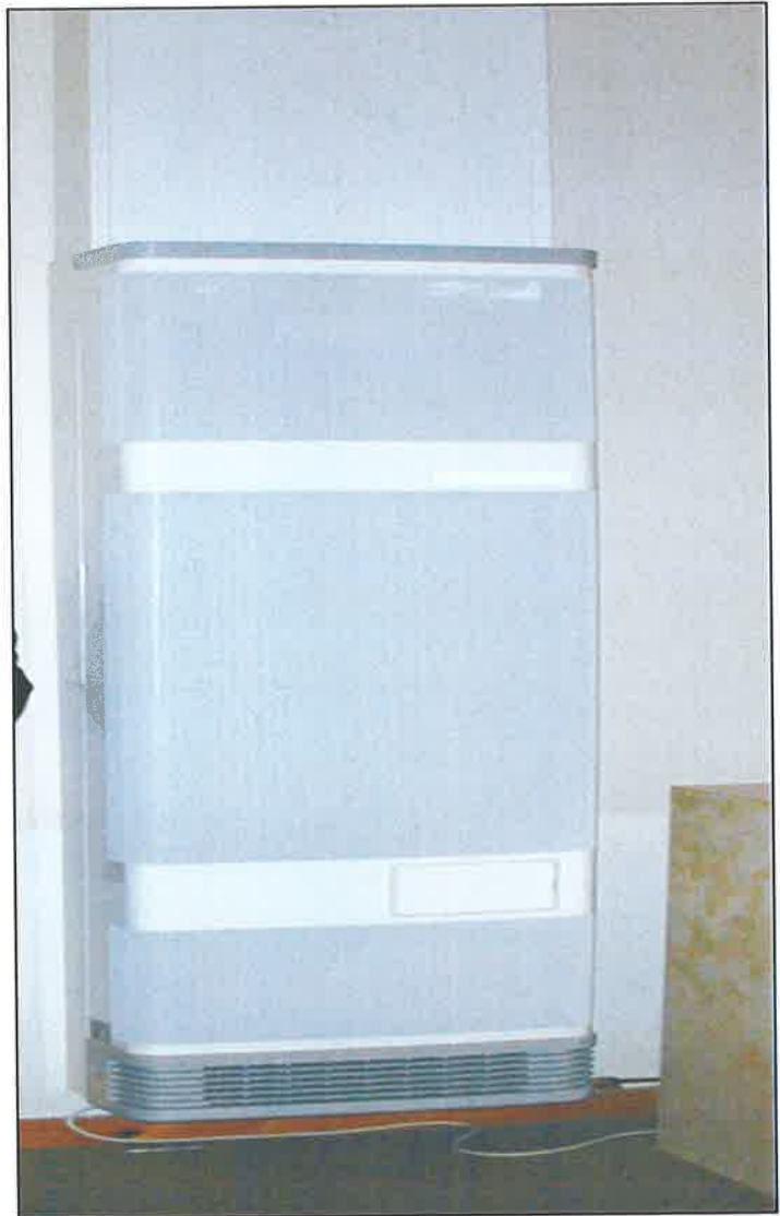
Flued gas replacement heater
