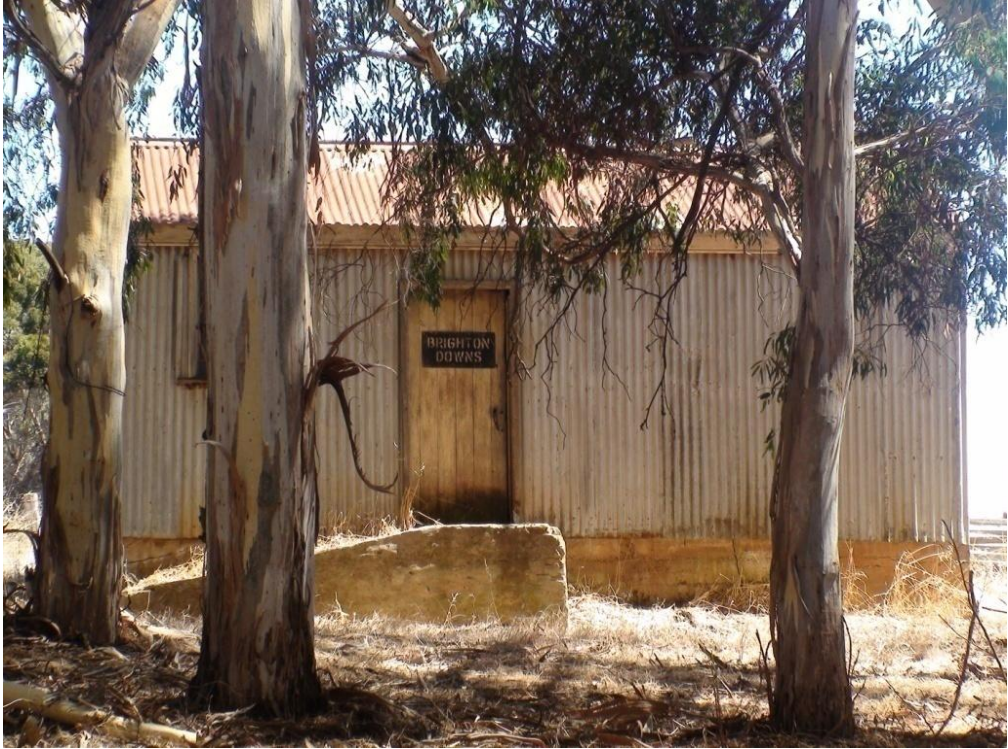
Figure 3.5 – Image of house and property name Brighton Downs (source: the author 2009)
