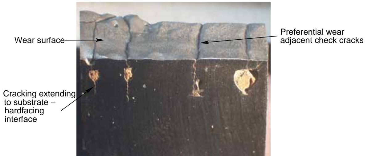
Figure 4.11: Cross section and wear surface of WeldoverlayB showing the check cracks extending to the substrate. Traces of slurry constituents can be seen in the check cracks and preferential wear adjacent the check cracks on the wear surface.
