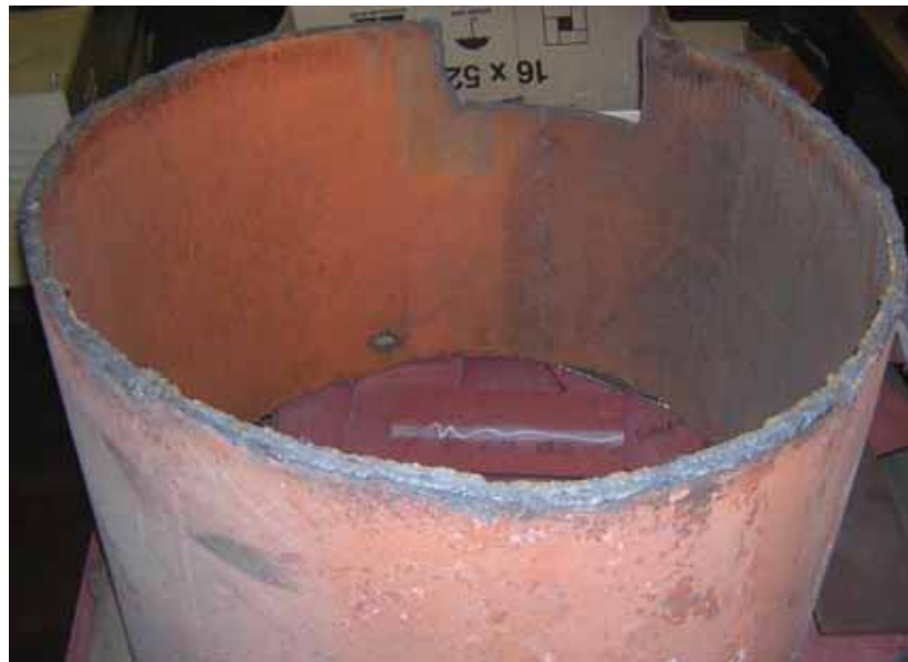
Figure 4.5: Overview of the ex-service alumina plant spool section designated as WeldoverlayA. Inside diameter of spool is approximately 725 mm. The rectangular cut out is the sample location.
