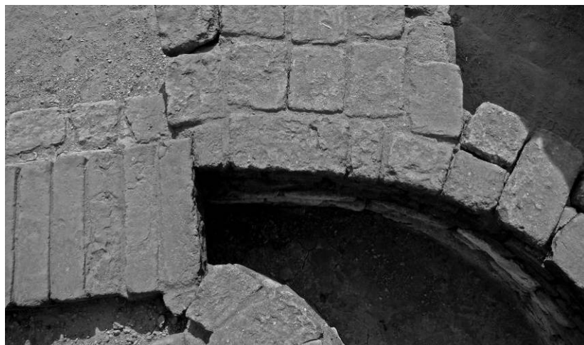
Fig. 7.45c. Detail of brick wall, Lothal, Gujarat. (Source: Photograph by author, 2007.)
