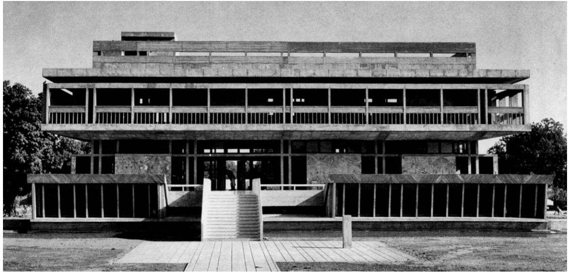
Fig. 7.37. L.D. Institute of Indology, Ahmedabad, India, architect B.V. Doshi. (Source: Curtis, Balkrishna Doshi: An Architecture for India , 16)
