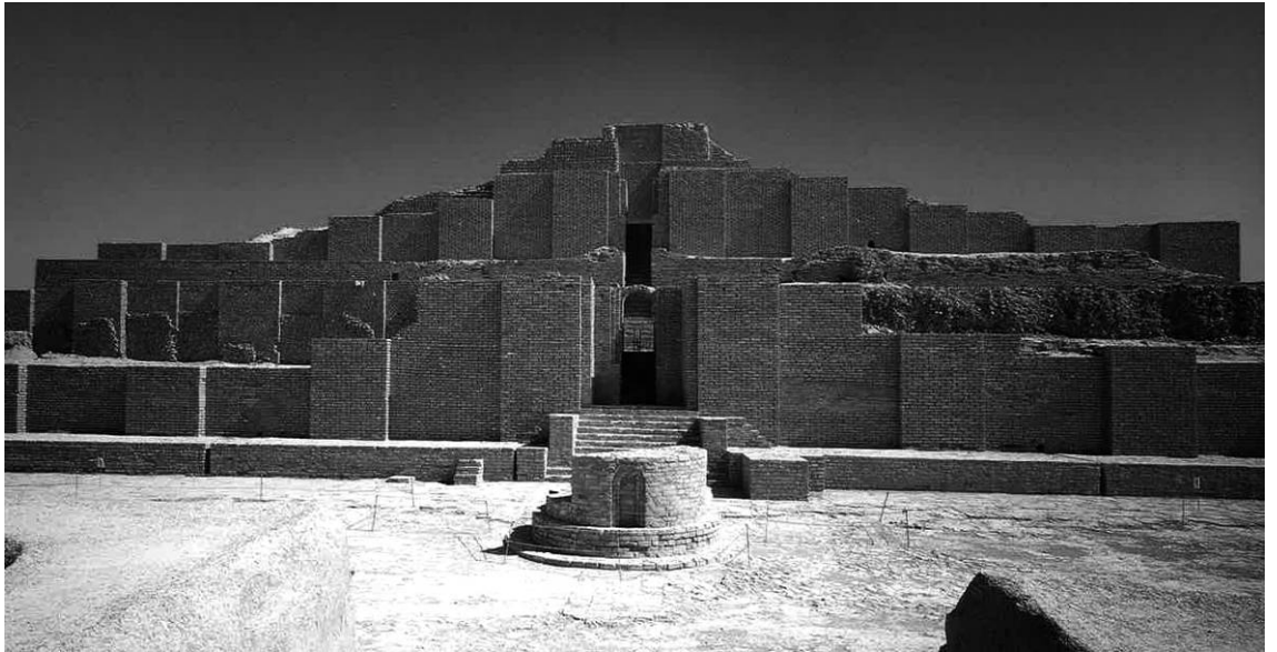
Fig. 6.5. The Ziggurat at Al-Untesh-Napirisha. (Source: Campbell, Brick: A World History , 32.)
