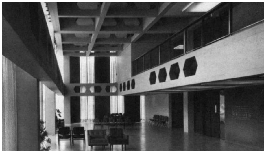
Fig. 7.53. Interior view showing vierendeel girders used for services, AFL-CIO Building. (Source: Leslie, Louis I. Kahn , 108.)
