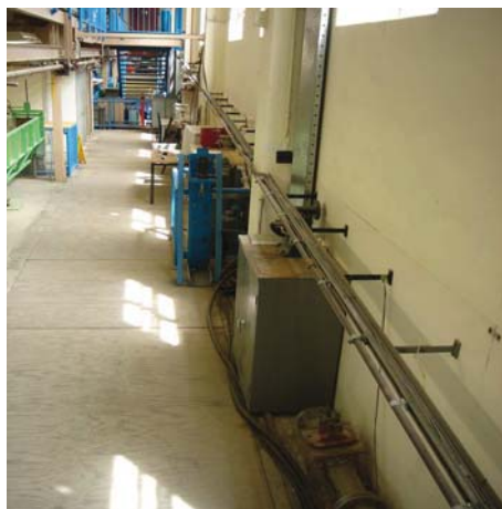
(c) The Middle of Pipeline
