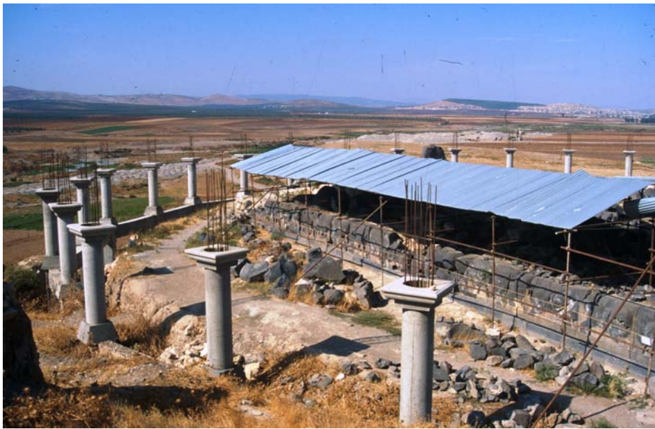
Fig. 11. Ain Dara: the proximity of the new concrete columns to the ruins. (Author: 1998)
