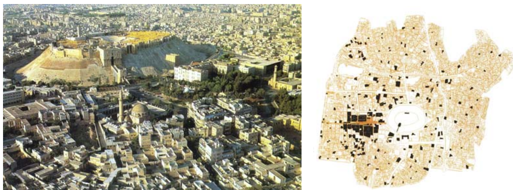
Fig. 21. Aleppo: an aerial view showing the Citadel and the close-knit fabric of the old city. Postcard from Aleppo, no date.
