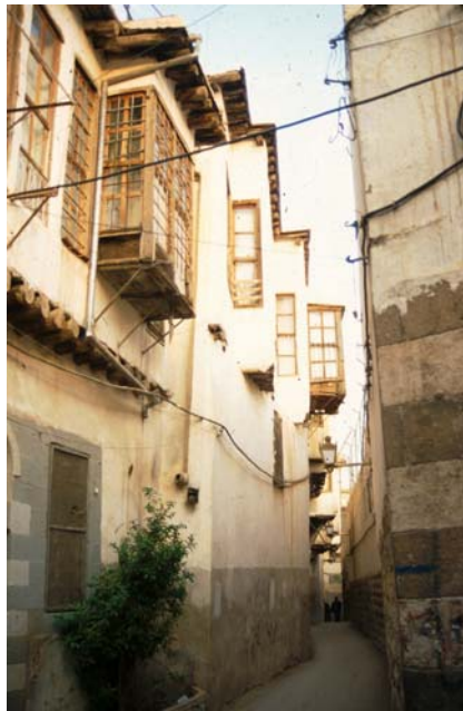
Fig. 55. Damascus: a street in the Old City. The Ottoman building on the right sits comfortably with later buildings in the rest of the street. (Author: 2002)
