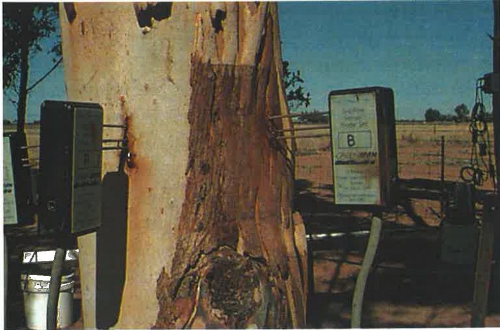
Figure 39 Heat pulse sap flow sensors installed in a tree at the water balance site.
