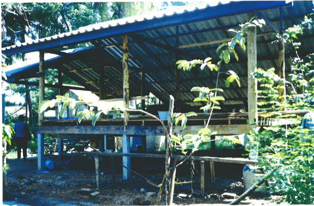
A. Houses that are under construction
