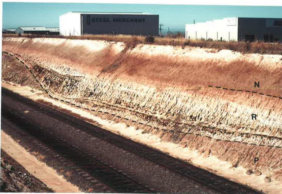
Figure 3.39 Quaternary sediments exposed in a railway cutting just south of O'Sullivan Beach Road. The Quaternary sediments fill a channel eroded into Precambrian sediments (P) with sands at the base assigned to the Robinson Point Formation (R) and reddish clays near the top of the sequence assigned to the Ngaltinga Formation (N). Basal sands are often mottled with iron oxides and bedding, which is highlighted by thin indurated intervals, is trough-like and generally follows the outline of the channel. The section exposed is approximately 6 m thick.
