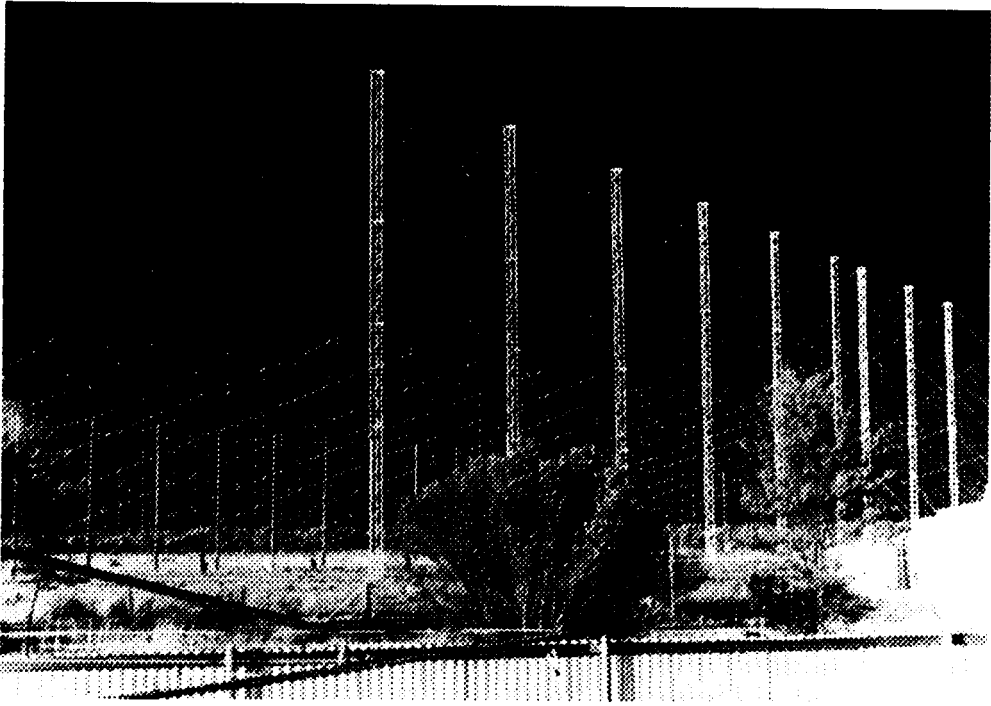
Figure 1.4: The Jindalee OTH radar transmitter site at Harts Range (100 km north-east of Alice Springs)
