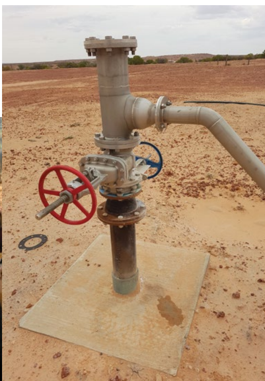
FIGURE 16 Uncontrolled open bore drain (left) and capped system (right). (Photos: L Brake & A Smith)
