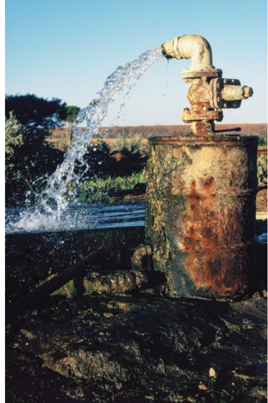
FIGURE 14 Flow from Beresford Railway Bore 1987, prior to capping. This well is no longer uncontrolled and was decommissioned in 2011 (Photo: C Harris)
