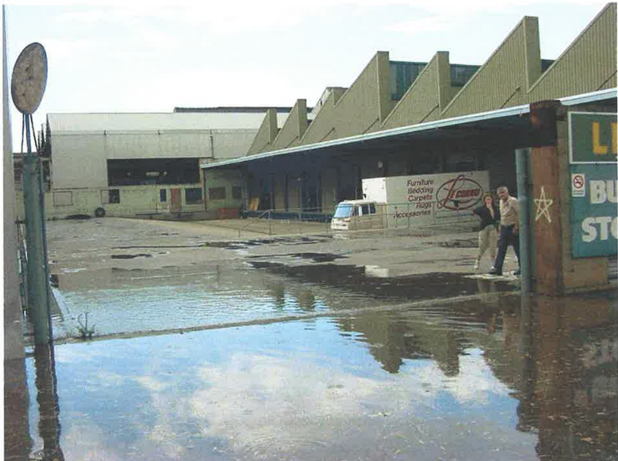
Figure C.4 Floodwater at the the gates of Le Cornu warehouse, 25 January 2001
