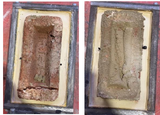
(ii) – Failed joint interface
