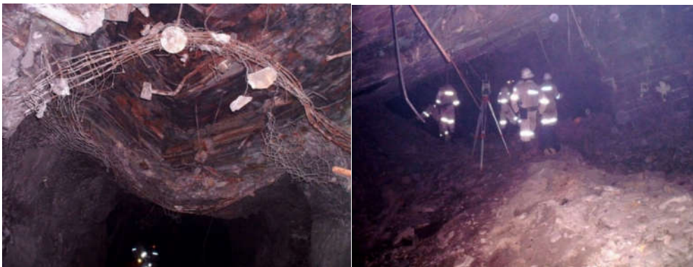
Figure 2-1. Squeezing in a tunnel at the NUG: (a) Crown sagging and (b) Floor heaving (Photos taken by the author).
