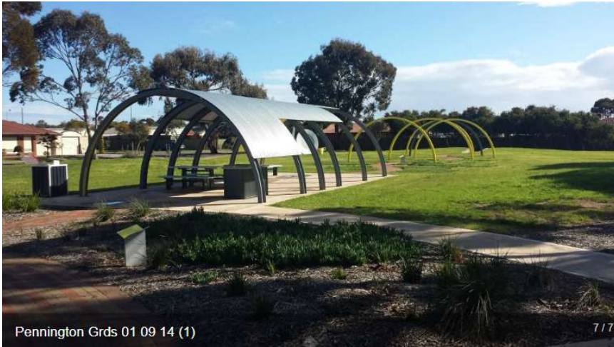
Figure 3: The Nissen hut-inspired barbecue shelter at the Pennington Gardens Reserve. Photo provided by the City of Charles Sturt.
