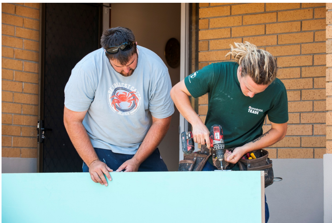
Matthew (left) and Kody (right) on work experience with Bettio Builders
