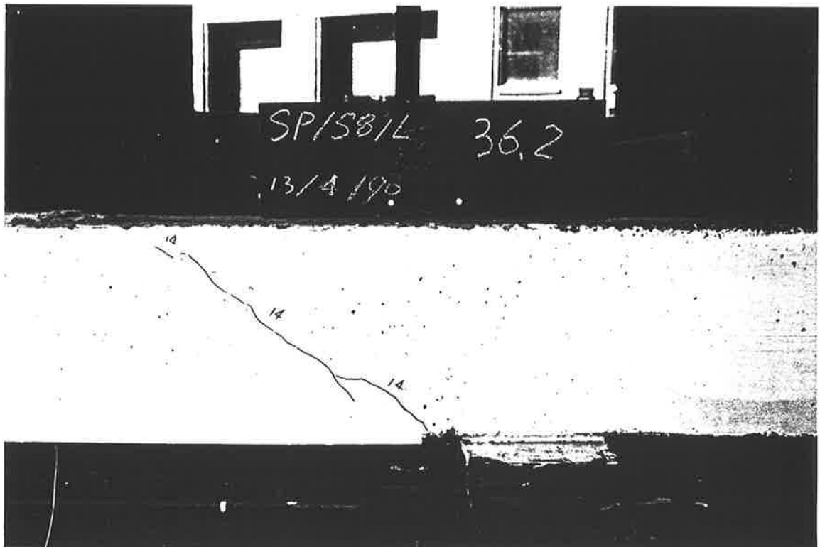
P3-53 The inclined crack formed
