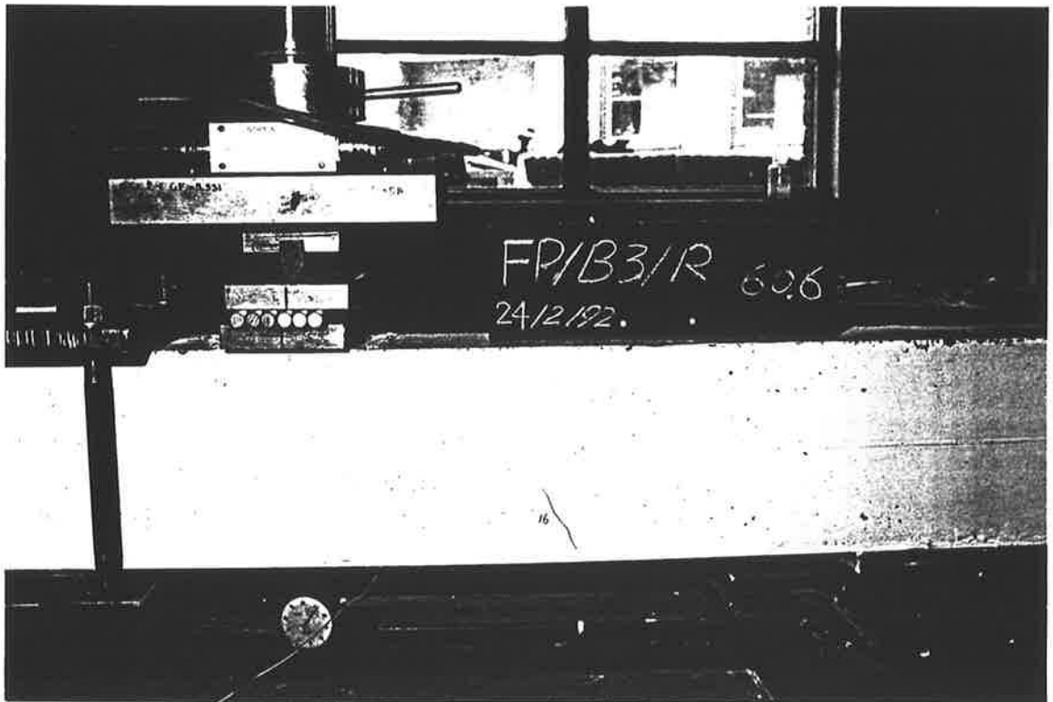
P3-41 The inclined crack formed
