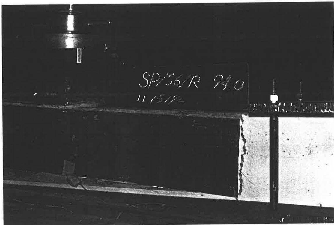
P3-79 The beam failed eventually in flexure
