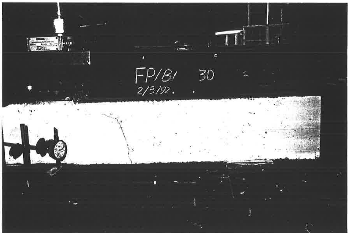
P3-28 Crack extended toward a point of the applied load
