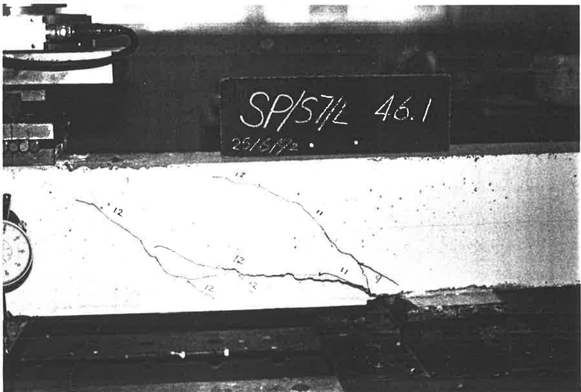
P3-82 Debonding of the soffit plate occurred
