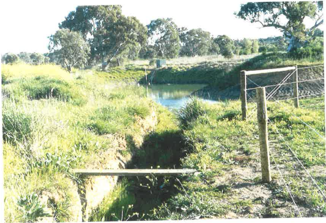
Photo 4.2 Off-take Diversion Channel
