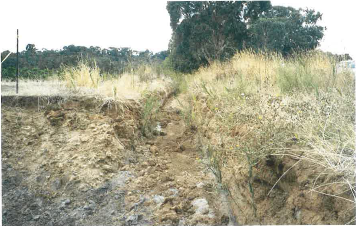
Photo 4.5 Off Stream Diversion Channel at Inlet to Storage
