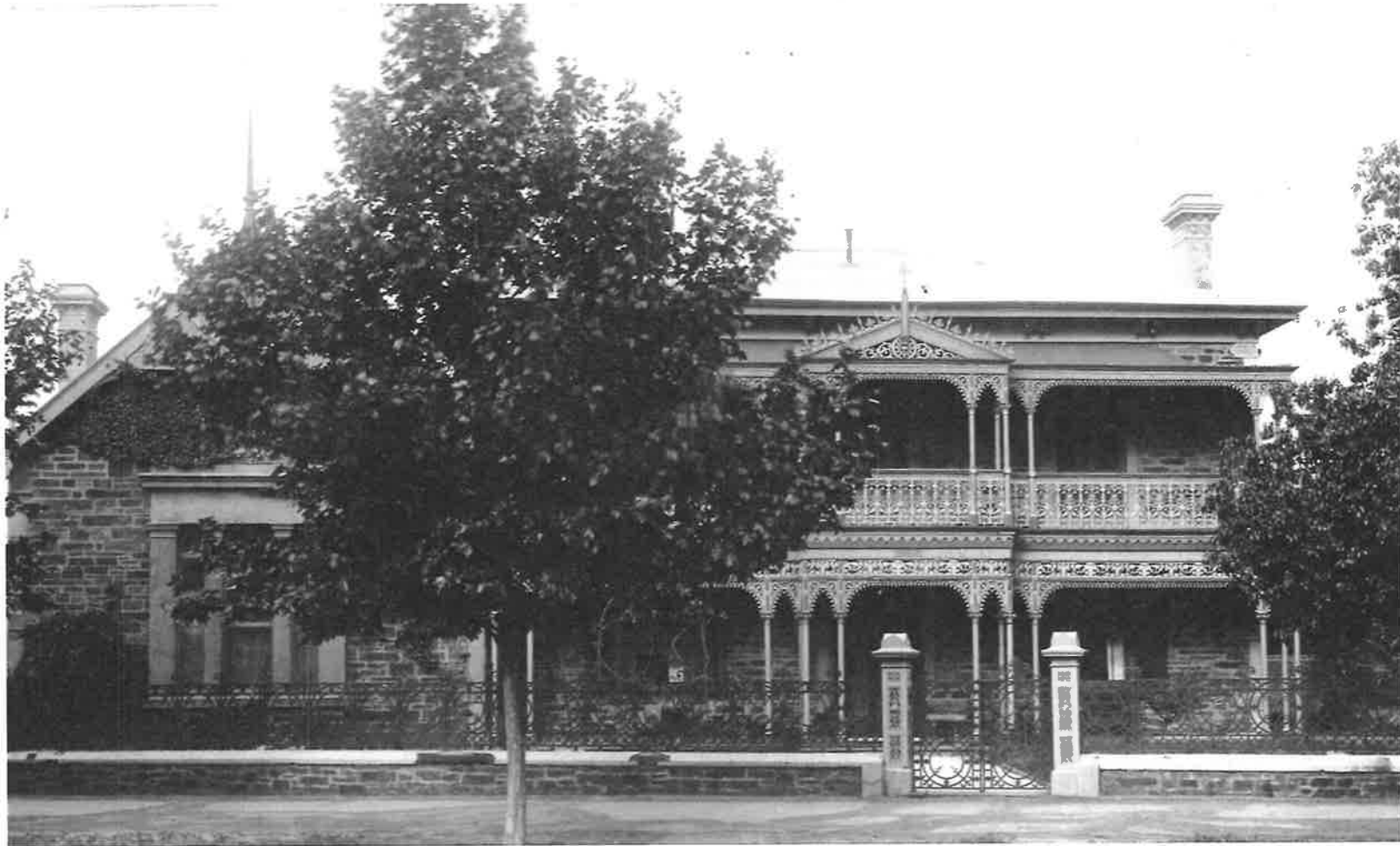
Royal British Nurses' Association headquarters, Dequetteville Tce, Kent Town, 1912. The building still stands. RAH Archives.
