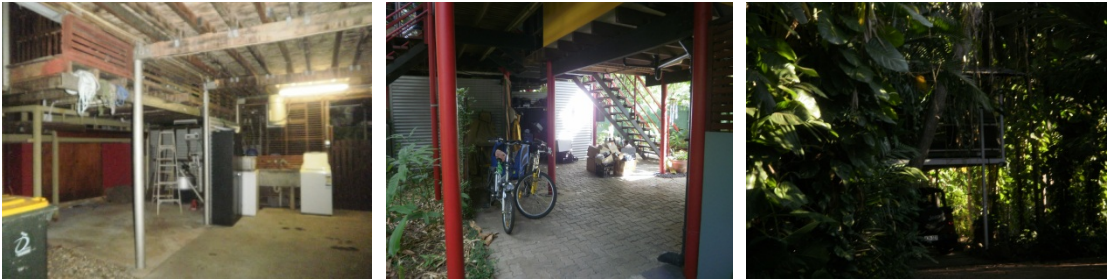
Figure 4.5.2m The under house space created by an elevated structure is used for parking, storage and an alternative way of outdoor living in the Lyne House (left), Kaiplinger House (middle) and Lyne House (right). Taken in 2011.
