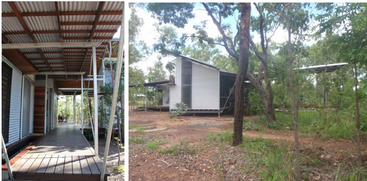
Figure 5.3.1a Prominent roof line covers an open breezeway (Left) as an invitation. It expresses the horizontality and the continuity of the sky-line. A strip of translucent window (Right) intersects the horizontality of a visually continuous verandah with the subtlety of verticality creating the unity of the sky and the ground as a whole. Taken in 2011.
