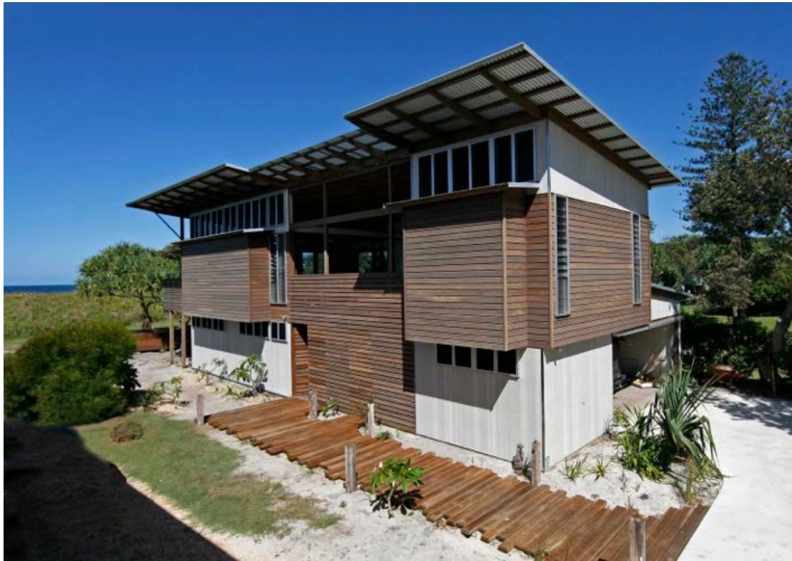
Figure 5.6.1b The Hutchinson Residence exhibits a hybrid style of Troppo house with key features of the 1980s Troppo houses and a symbolic expression of modern living
