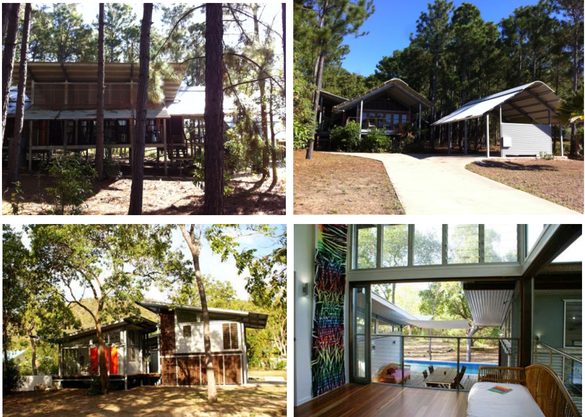
Figure 5.4d Two Horseshoe Bay residences were built on Magnetic Island between 2006 and 2010. They display the characteristics of an elevated lightweight structure, complete exposure and openness to nature through windows, doors, louvers and translucent polycarbonate cladding sheeting (Top Left and Right photos taken by Huang, July 2012. Bottom Left and Right photos taken from the website of Australia Institute of Architects for competitions in 2010).
