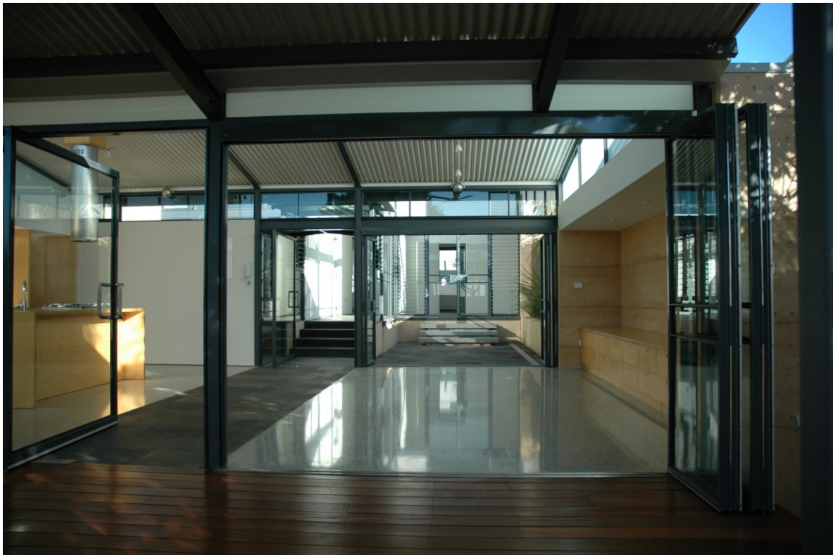
Figure 5.7b This house was initially chosen for the final case study of Troppo house in Perth but replaced due to some foreseen difficulties. Nevertheless, an open plan offers a natural air-flow with the assistance of ceiling fans and glass louvers. The post-and-beam steel frame, an open indoor-courtyard, and exposed corrugated-iron roofs retrospect the early design of Darwin Troppo houses. Thick rammed earth walls and cool marble floors are used in response to Perth's winter.
