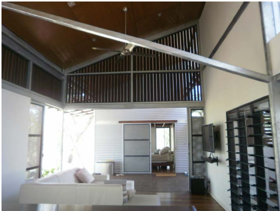
Figure 5.3.1j The double-height spaces in the verandah (Top) and living room (Bottom) give a sense of awe and spaciousness. The transparency of living areas is given by minimizing the solid external walls with large sliding doors, glass louvres and timber strips.
