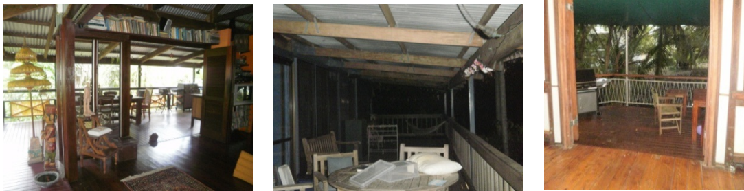
Figure 4.5.2l Verandahs are used as open outdoor living spaces. They are extendable spaces of the living room and of the bedroom. Their multi-functional purposes are apparent in the Kaiplinger House (Left), Green Can House (Middle), and Troppo House (Right). Taken in 2011.
