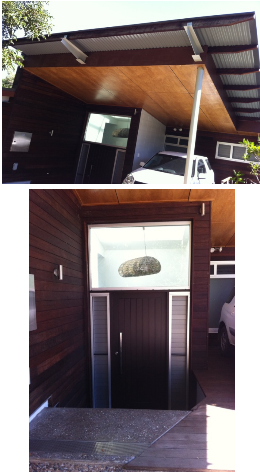
Figure 5.4.1i Covered timber ceiling with soffit and fascia (Top), polished concrete floor and aluminium fixed-framed windows (Bottom).
