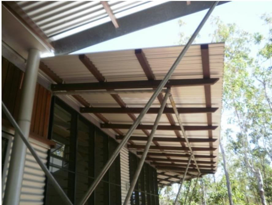
Figure 5.3.1b Compared with Troppo's 1980s Darwin houses, there are resemblances of design elements such as corrugated iron panels for walls and roof, glass louvres, timber deck, posts, and floor in the Mortlock Residence with a new feature – metal poles for supporting long timber structure overhangs (Top) which are connected to the main steel structural framework of the house (Bottom).
