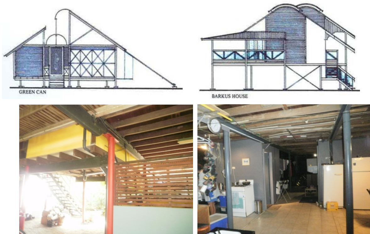
Figure 6.3.2. The elevations of the 1980s Darwin houses show steel cross-bracing members. The photographs show the intentional short-span of floor joists, bigger size circular hollow sections (CHS) and I-Beams, and unseen deeper footings (on the bottom row) as 'over-engineering' structures for assuring the occupants of the structural durability and stability in case of any cyclones and flood.
