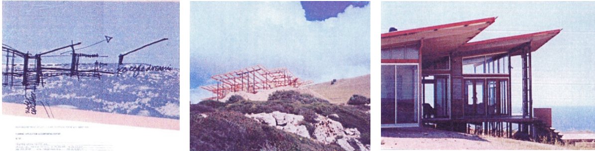
Figure 4.4.5 Harris' on-site sketches (Left) drawn in September 2000, the photo of the exposed timber framework of the house (Middle) taken in August 2002, and the photo of the completion of the Cape du Voltigeur House (Right) taken in December 2003 perched on a ledge of Kangaroo Island, South Australia.
