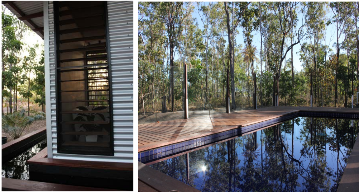
Figure 5.3.1c Exclusively new design elements are the water box around the bathroom (Left), timber louvres, plastic translucent roof sheeting, angled posts, the steel cross-brassing on the windows, and minimum areas of construction materials meeting the ground. An element of nature – water – suggests a calm and peaceful place outside bustling urban city life of Darwin with a pool (Right).
