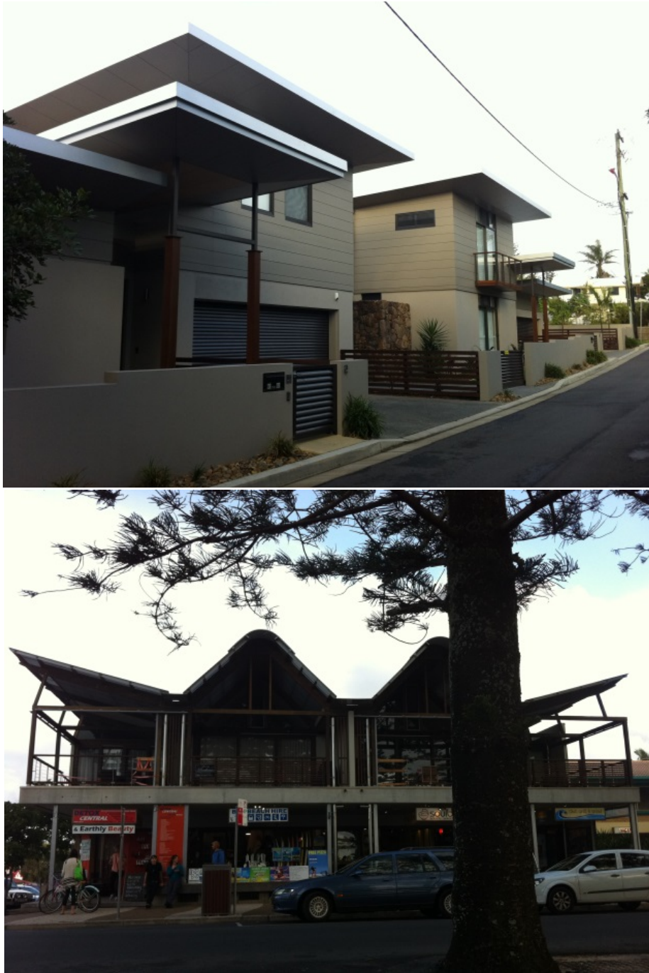
Figure 5.6c The contemporary Troppo language in grouped townhouse (Top) designed by Troppo's Byron Bay office in the 2011 and a mixed-use accommodation and retail building (Bottom) collaboratively designed by both Troppo's Byron Bay and Adelaide offices in the central area of Byron Bay. This mixed use building was built in 2004 and received the Grand Winner and Award for Excellence for Northern Rivers Urban Design Awards in 2008.
