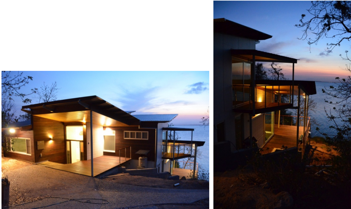
Figure 5.4.1a The Connell Residence is situated on the rocky cliff side of Northern Magnetic Island (original photographs taken by Khamisa after the completion of Connell Residence in 2012).
