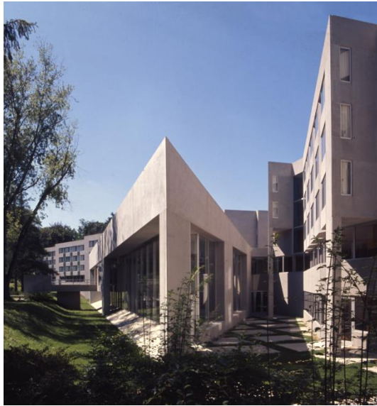
Figure 2.10 Mission Park Residential Houses, Williams College, 1972. Courtesy of The Architectural Archives, University of Pennsylvania. Ref: aap.267.144.13_a
