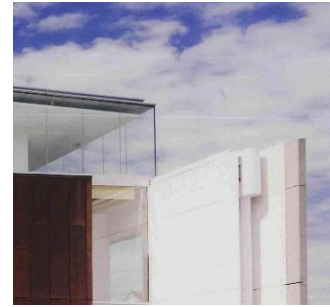
Figure 6.30: Detail of St Patrick's floating screen wall. Photograph by author.
