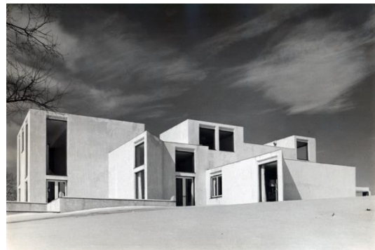
Figure 4.28: White Residence, 1963. Courtesy of The Architectural Archives, University of Pennsylvania. Ref: aaup.015.V.131.1
