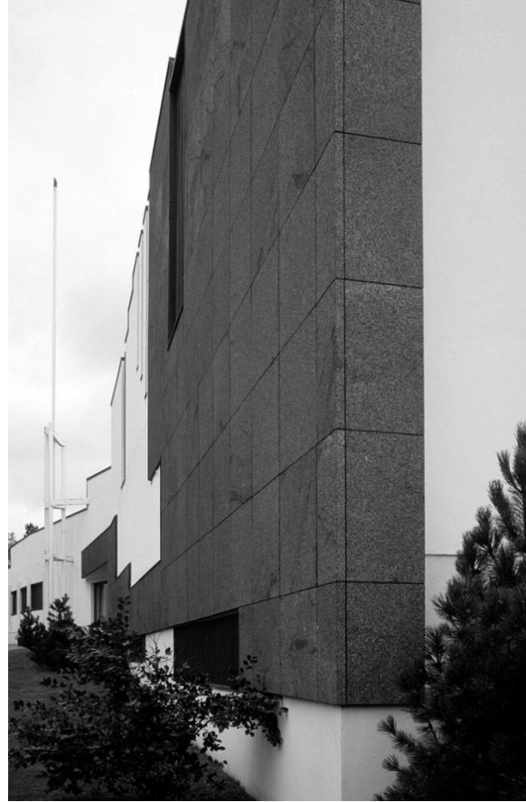
Figure 4.30: Detail of Alajärvi Town Hall, 1966, Alvar Aalto, showing the irregular overlay of stone veneers. Photograph by Josep Maria Torra (2008). CC BY-SA 3.0.
