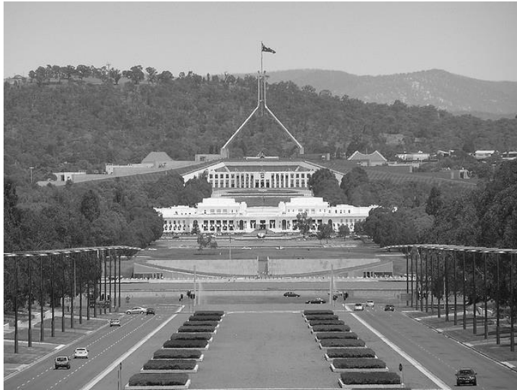
Figure 4.23: View of Parliament House from War Memorial Drive. Photograph by Max Jefferies.
