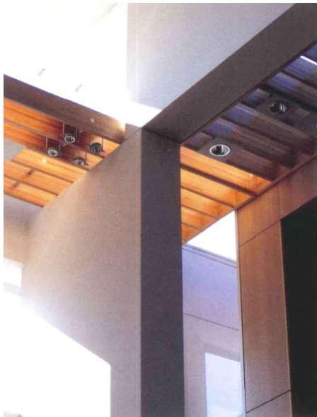
Figure 6.33: Junction of blade wall and roof beam. Photograph by Hamilton Lund. Reproduced with permission from Luminous Simplicity: The Architecture and Art of St. Patrick's Cathedral, Parramatta . (Giurgola 2006:83)
