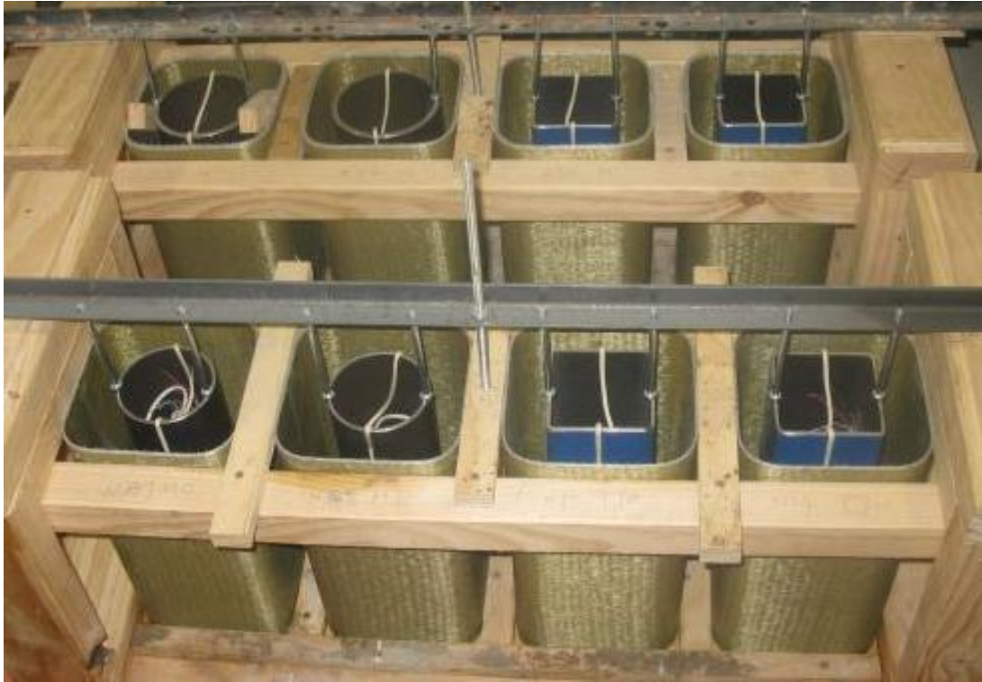
Figure 2. Formwork used in fabrication of DSTCs
