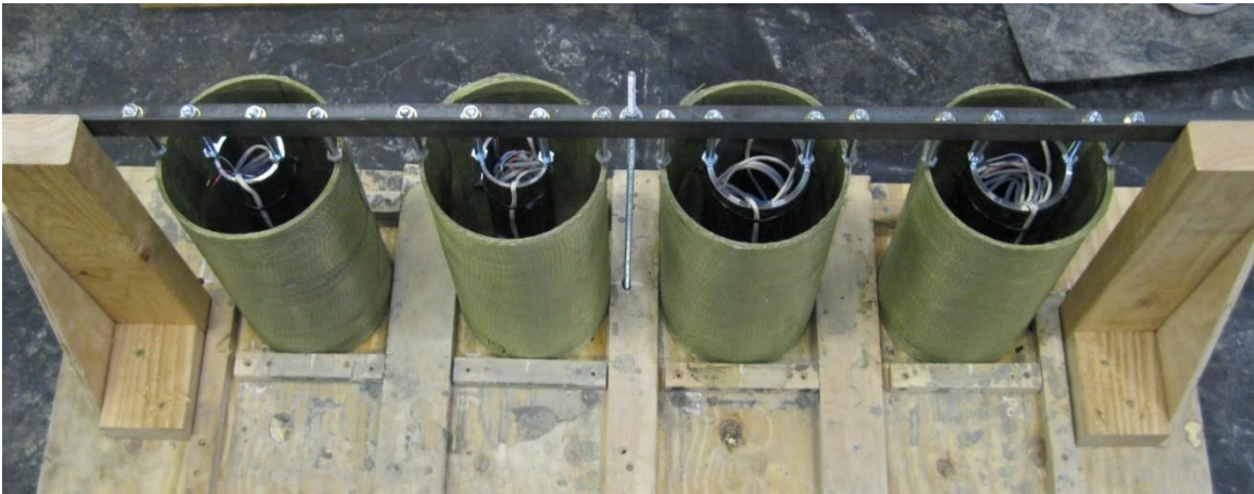
Figure 2. DSTC specimens before concrete pouring
