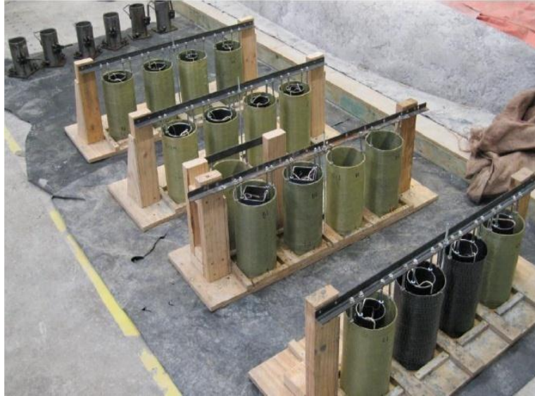
Figure 1. DSTC specimens before concrete pouring
